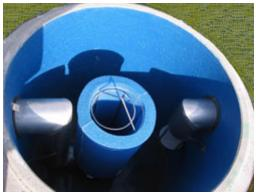
Since the inside of the separator should be periodically inspected and cleaned, it is advisable to locate the unit outside any roads, parking lots, etc. Location of the unit should allow easy access of the vacuum trucks for performance of maintenance work.
